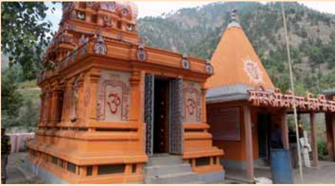
Ramban Saraswati Mandir Jammu & Kashmir constructed by Kanchi Kamakoti Peetham
